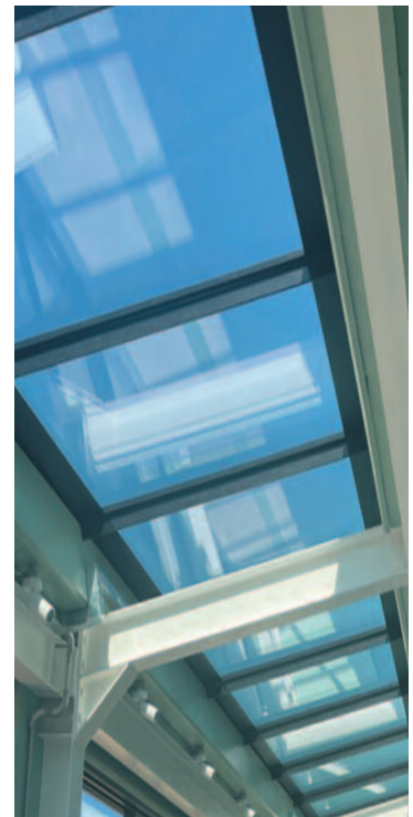
Large roof window incorporated into the middle of an Infinity solar roof.
